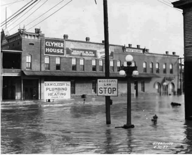
FIGURE 8.2 Downtown Greenville, Mississippi, on April 30, 1927, six days after the levee break. (Photo courtesy of the Mississippi Department of Archives and History.)
